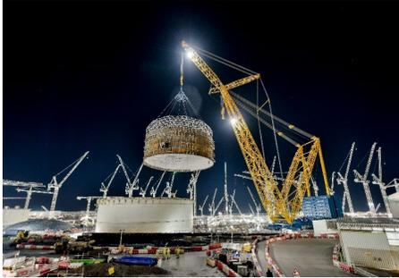
Big Carl, the world's largest crane, has just completed its biggest ever lift at Hinkley Point C. The super-crane lifted a total weight of 575 tonnes to install the first of three massive, prefabricated steel rings which form the reinforced cylinder around the nuclear reactor.
