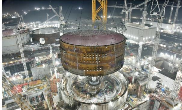
This “replication effect” will benefit the identical Sizewell C project in Suffolk. The prefabricated ring, which is 47 metres in diameter and 17 metres high forms a reinforced cylinder around the nuclear reactor and is a key milestone in the construction of the second reactor building.
