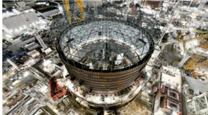
The 347-tonne lift takes the structure to a height of 32m and means that just one more liner ring is needed before the dome roof is lifted into place.
