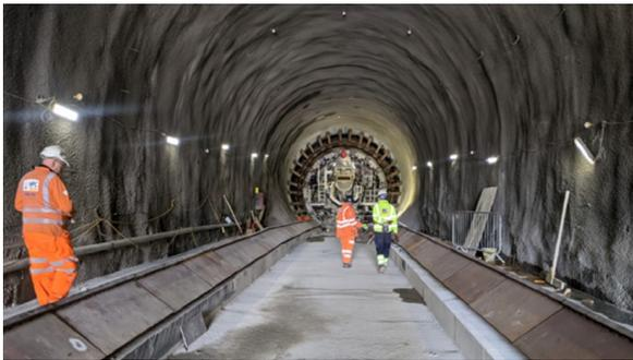
Beatrice, the site's third Tunnel Boring Machine (TBM), has successfully completed the main drive for intake tunnel two, a key milestone for the project. This follows previous journeys taken on intake tunnel one and the outfall tunnel by TBMs Mary and Emmeline respectively.
