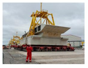
The first 5,000 tonne cooling-water intake heads were carefully loaded onto barges at Bristol Port's Avonmouth docks, ready to be towed out to meet two floating heavy lift cranes off HPC – Rambiz and Gulliver. The four "intake" and two "outfall" heads have been built by Balfour Beatty in Avonmouth. Each "loading out" operation, carried out by lifting specialists Mammoet, takes several hours, with the water levels being adjusted at the dock, to ensure the
