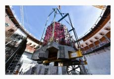
Big Carl was also kept busy lifting the second of four accumulator tanks into position in the northeast corner of the Unit 1 reactor building. The accumulators are an essential safety component that will kick into life supplying coolant to the primary circuit in case of a loss-of-coolant incident and without the need for outside intervention. The huge tank weighs in at around 50 tonnes and measures at 9.1m tall by 3.5m in diameter.
