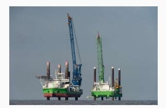
This is what will eventually allow seawater to pass through into the power station. The first step will see the casings hammered into the seabed in each of the six head locations. Then, mining operations will take place to create a socket for the liners to be positioned into. The liners have been specially designed and fabricated in Scotland and each one weighs more than 270 tonnes (more details below).
