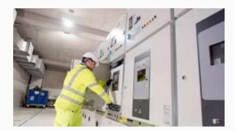
The 10kV switchboards distribute electrical power to essential equipment such as the reactor cooling pumps, as well as to lower voltage equipment. Their installation and eventual energisation will enable the commissioning of the rest of the plant's electrical infrastructure.
