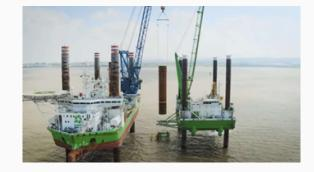
These 5,000-tonne structures were lowered onto the seabed last year and will circulate water to the nuclear reactors.
